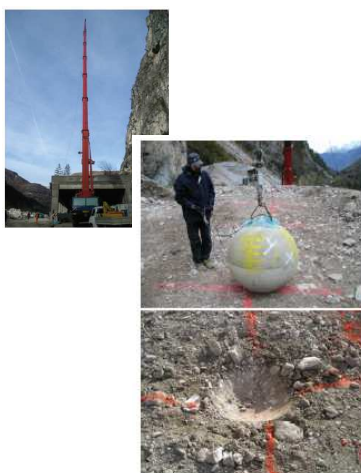
Protection against rockfall: boulder impact test on sheltering structure
