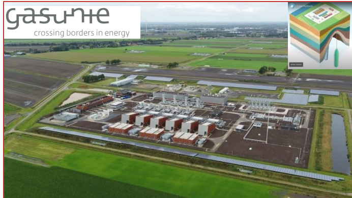
NL: UHS in Salt Caverns, Zuidwending
