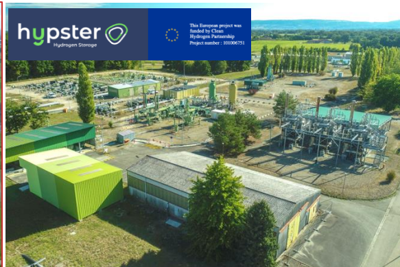
France: UHS in Cavern, Etrez
