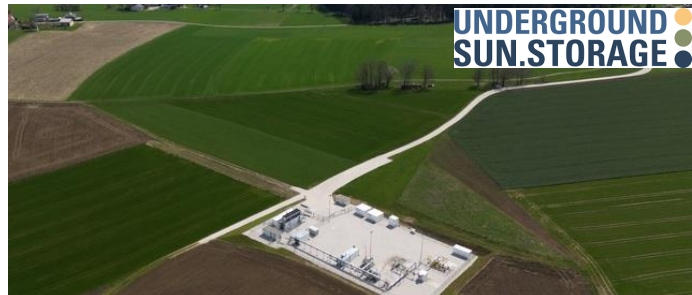
Austria: UHS in Gas Field, 2023 (RAG)
